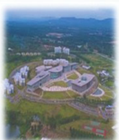
Facility Condition Audit @ AIMST University Building
