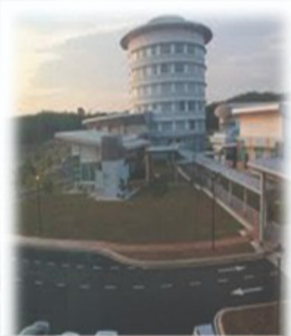
Facility Management Service @Akademi Kementerian Pengajian Tinggi (AKEPT), Enstek, Negeri Sembilan
