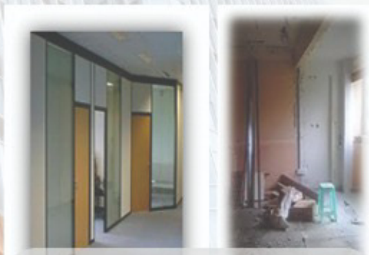
Interior Renovation works of Office Project @ Kamimaru (M) Sdn Bhd Kota Kemuning
