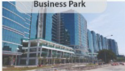
Menara UOA Business Park
