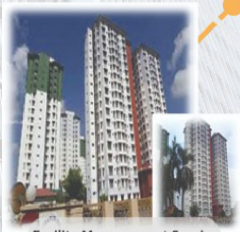
Facility Management Service @ Pangsapuri Ilham, TTDI Jaya, Shah Alam
